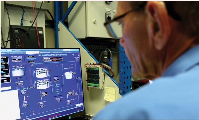
Water Services team member checking remote SCADA systems in Alice Springs.
